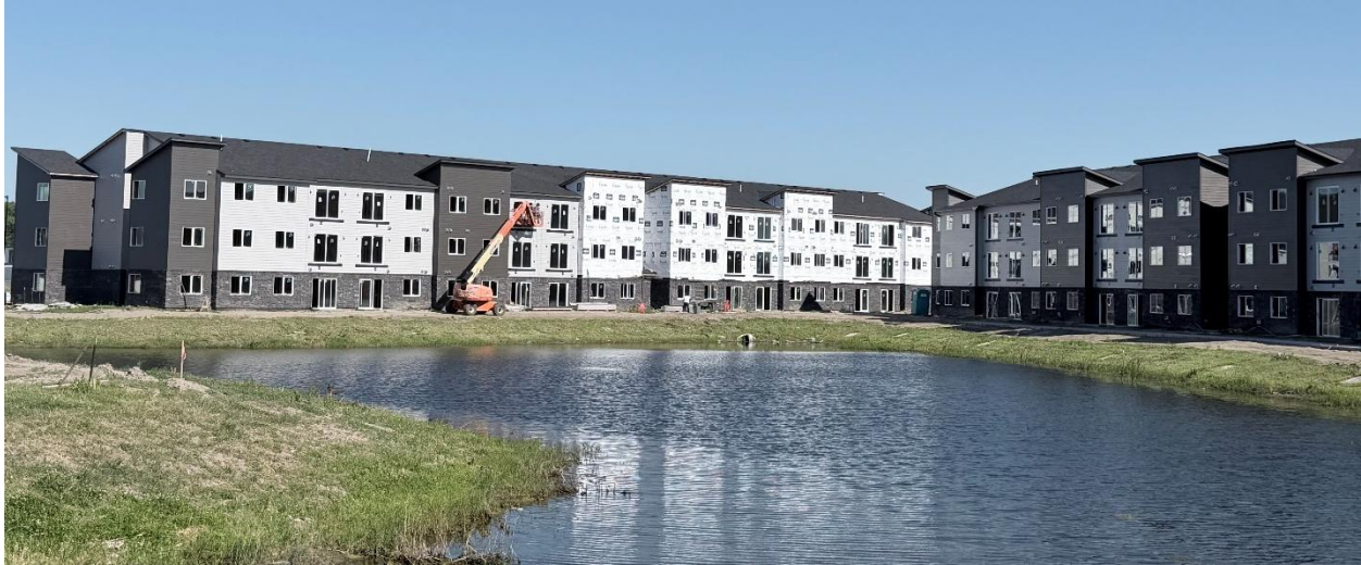
Figure 6.24: New Multifamily Housing Construction in Columbus, 2026
