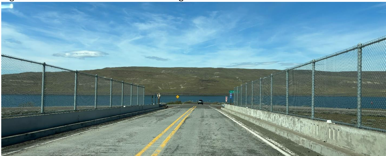
Figure 2.3: Willow Creek Site Access Bridge
