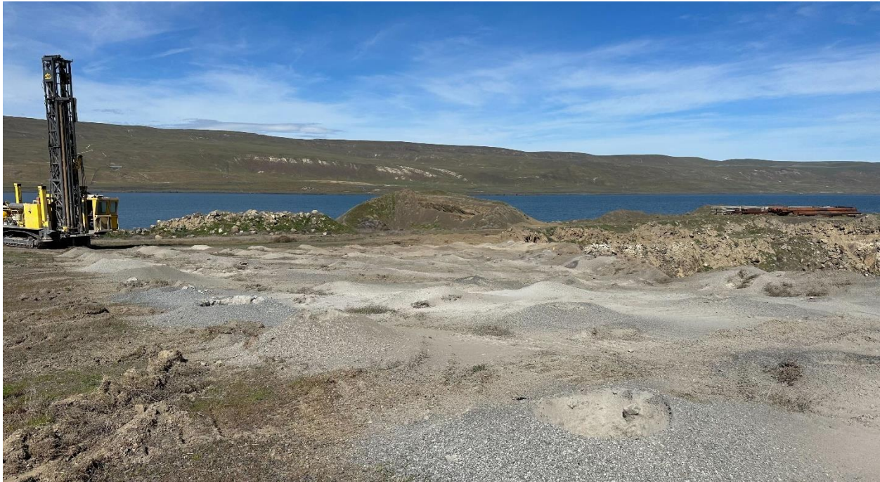
Figure 2.2: Willow Creek Site Gravel Quarry
