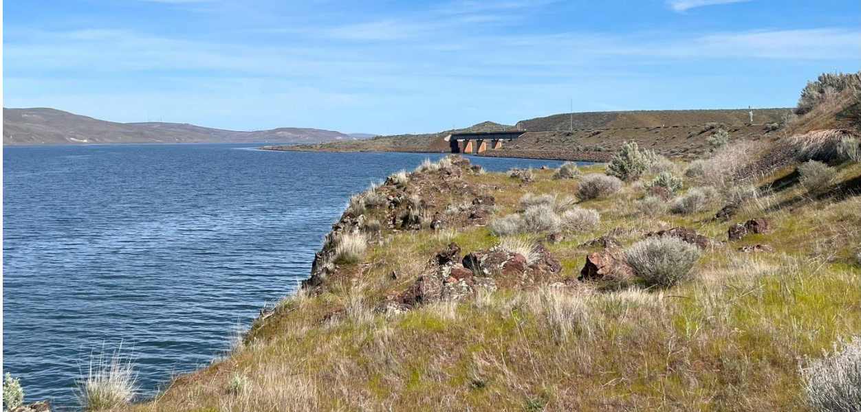
Source: Points Consulting, On-site Visit, April 2024
