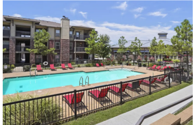
Figure 14: Pool at ‘The Icon at Broken Arrow’ apartments
