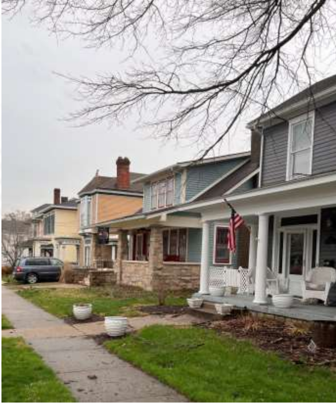
West 4 th Street in Frankfort (Special Capital District) has tighter average housing densities and hosts numerous duplexes and quadplexes
